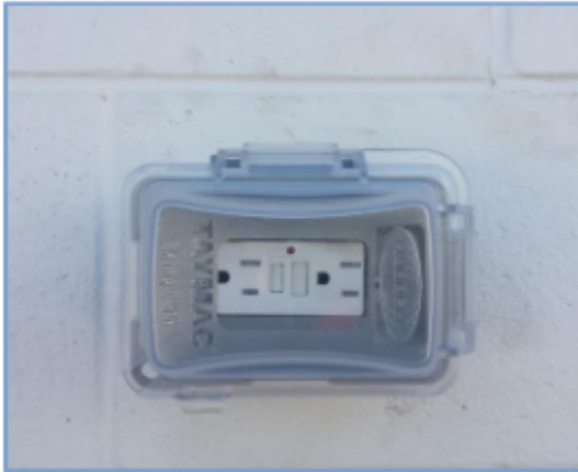
(Example of GFCI outdoor rated outlet with cover)
