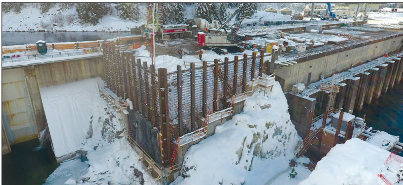
Construction of the Upstream Fish Passage at Box Canyon Dam
