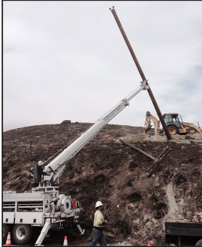
PUD line crew rebuilding distribution line in Okanogan County
