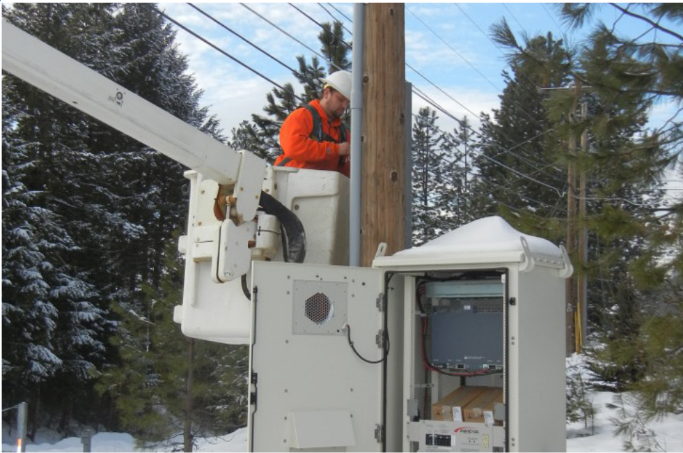
CNS Technician performing storm repair on fiber optic system.
