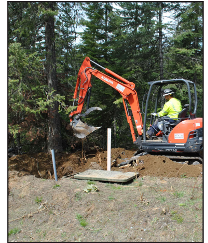
Underground fiber optic line installation
