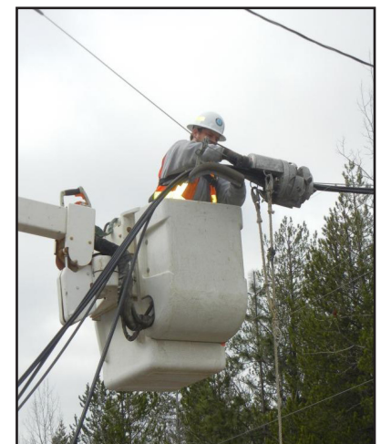
Overhead fiber optic installation work
