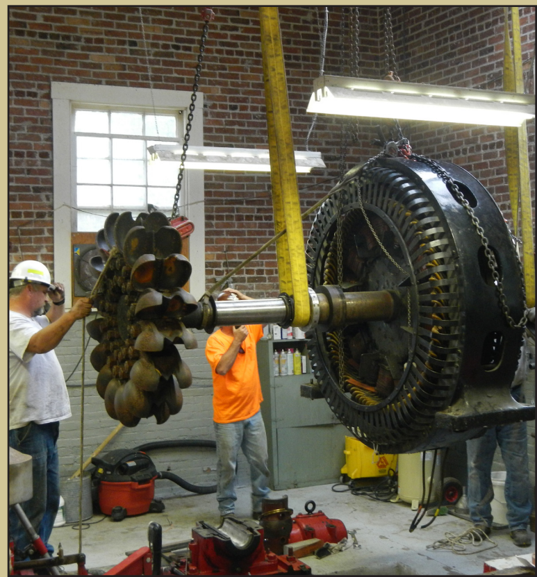
Calispell Creek Power House generator being lifted out of the powerhouse.
