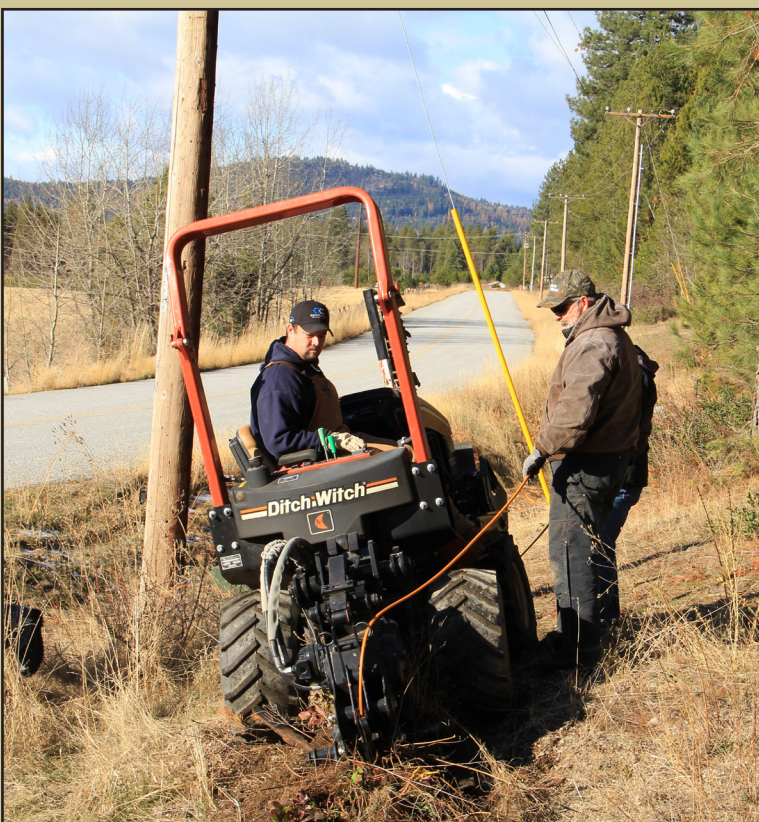
Mike Reed, CNS Technician plowing fiber optic service drop.
