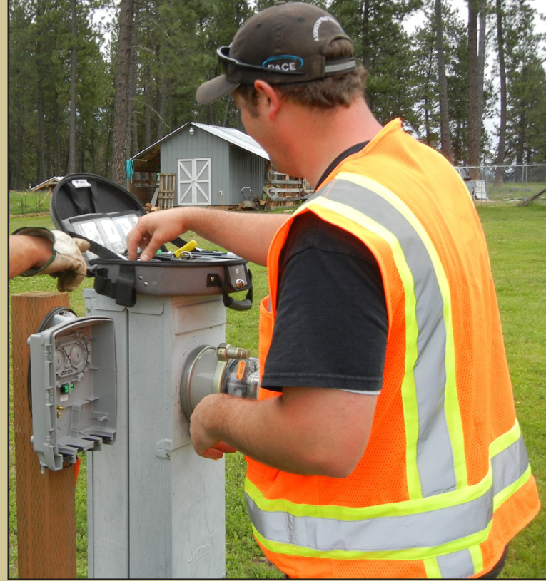
Patrick Barley, CNS Technician, installing fiber optic electronics.
